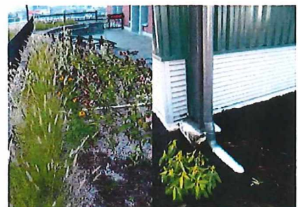
A rain garden is an attractive way to manage polluted runoff on site. Photo: Erica Guttman
